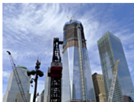
Freedom Tower, center, rising at Ground Zero in Lower Manhattan, September 2011
